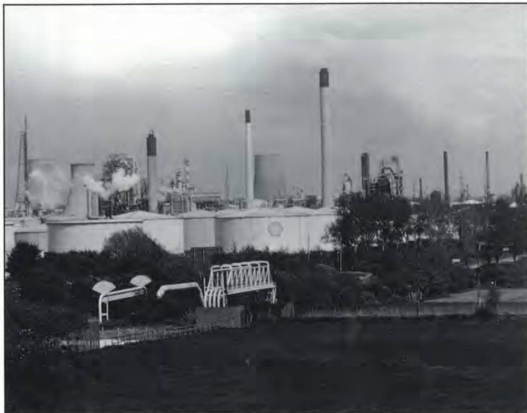
Cheshire Region includes major industrial customers along the banks of the River Mersey.
